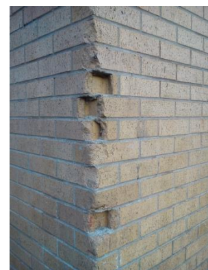
Figure 10: Deteriorating brick
