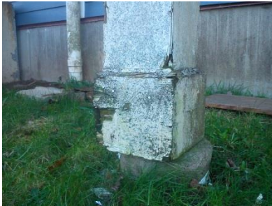
Figure 7: Deteriorated awning support
