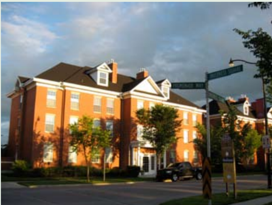
Figure 23: High end new urbanism housing product in McKenzie Towne, Calgary
