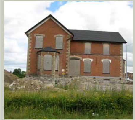
Figure 10: An old farm house makes way for new housing development along Markham’s ever-expanding borders (Katherine Perrott)
