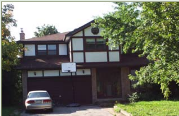
Figure 3: Single detached house built in the late 1970s in Markham (Joe Perrott)
