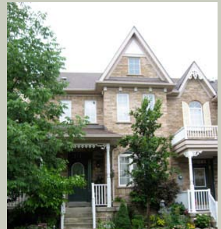
Figure 15: New urbanism's back lanes allow for attractive house facades without garages, creating desirable streetscapes (Katherine Perrott)
