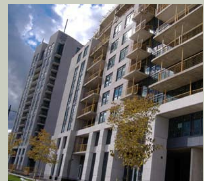
Figure 14: High Rise condominium in Markham Centre (Katherine Perrott)
